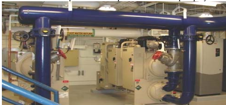
Figure 6 Large Temperature Difference Variable Flow Transmission
